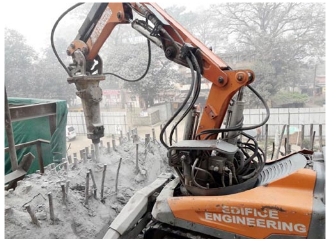
Photo 6: Salvaging of fly over structure
