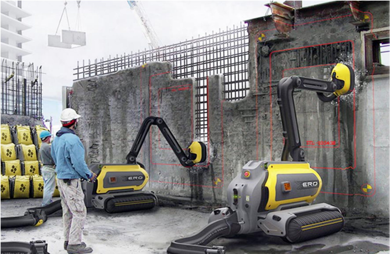
Photo 3: Robot for eating concrete
