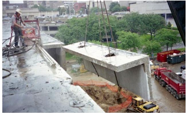
Photo 6: Salvaging of fly over structure
