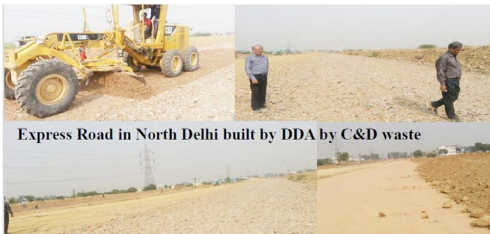
Photo 19: Road constructed with C&D waste processed material at Delhi
