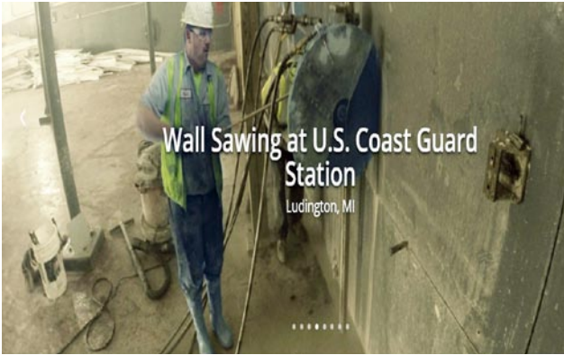
Photo 5: Sawing of wall
