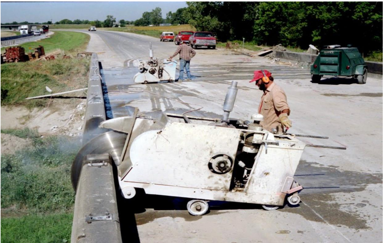
Photo 4: Salvaging of Parapet
