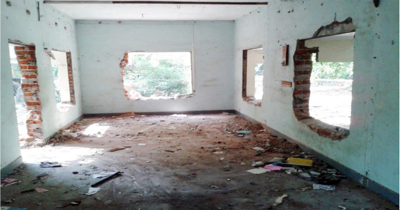
Photo 1: Salvaging doors and windows
